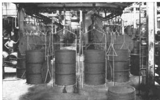
Port Arthur, Texas, Cleaning Line
