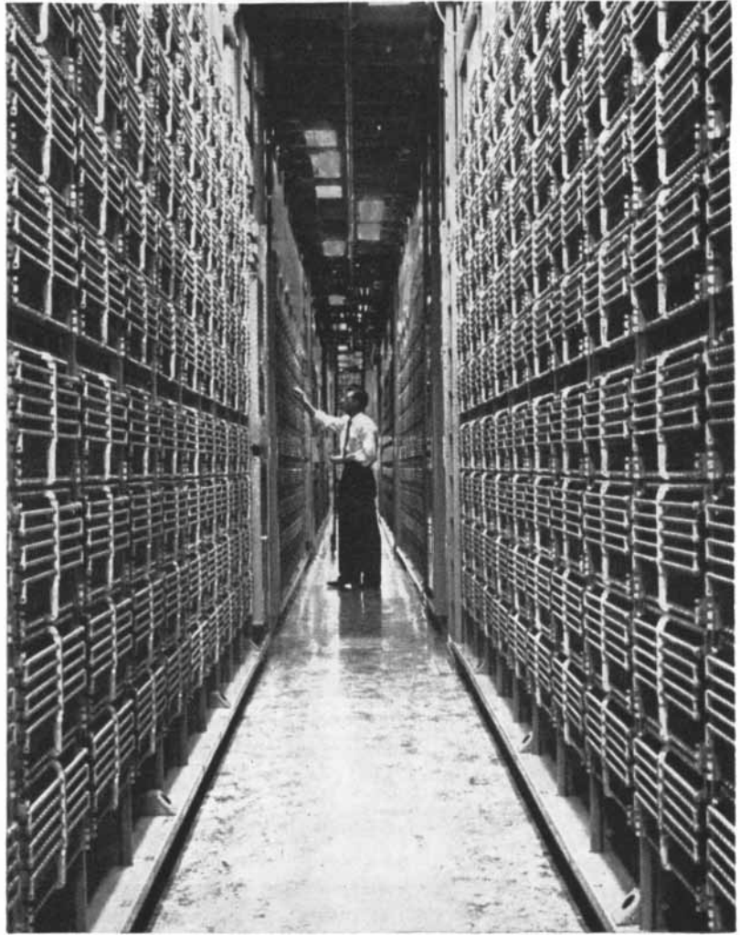
In a large, modern telephone office, two million relay contacts await the orders of your dial to clear a path for your voice. They open and close a billion times a day.
