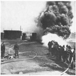
2. MILITARY FIRE-FIGHTERS need pumps that are easily portable, quick and dependable in operation. Latest development in this field is the portable gas turbine, now proving itself as a versatile power source. Fenwal Over-Heat Detectors, developed for the aircraft field, are the thermostatic units used to protect the new gas turbine against overheating.
