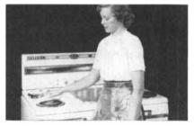
Sears-Roebuck's new Kenmore range with a Sylvania instant-heat lamp unit which has a VYCOR bulb and tinted cover plate.
