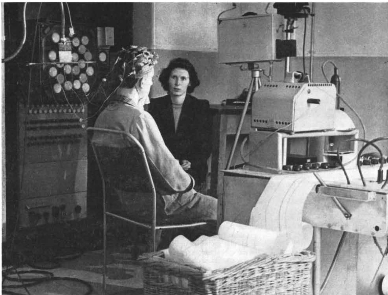
ELECTROENCEPHALOGRAM is made at the Burden Neurological Institute in Bristol, England. The electrodes are attached to the scalp of the subject, who is seated with an investigator. Where an
