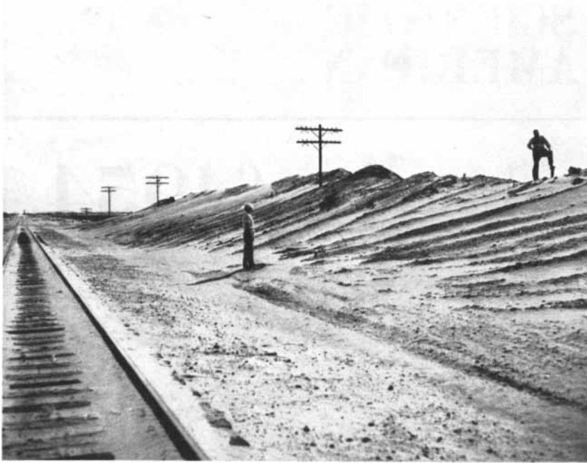
RAILROAD TRACKS on the border of Terry and Yoakum counties in West Texas were cleared of drifting soil before this photograph was made. Telephone poles are half buried.
