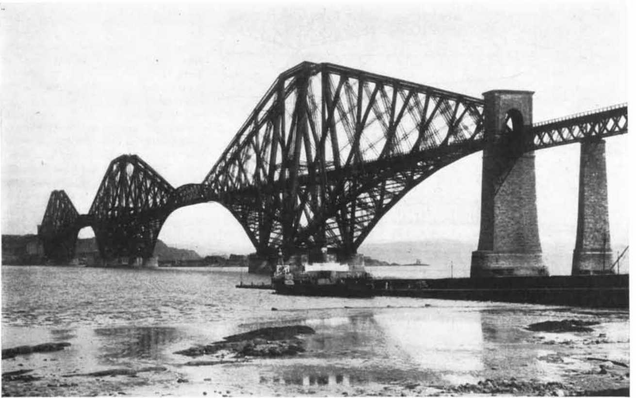
FIRTH OF FORTH BRIDGE in Scotland possesses two huge cantilever spans, each 1,700 feet long. These spans were the longest in the world from 1890 until 1917, when the Quebec Bridge across the St. Lawrence River surpassed them with a length of 1,800 feet.
