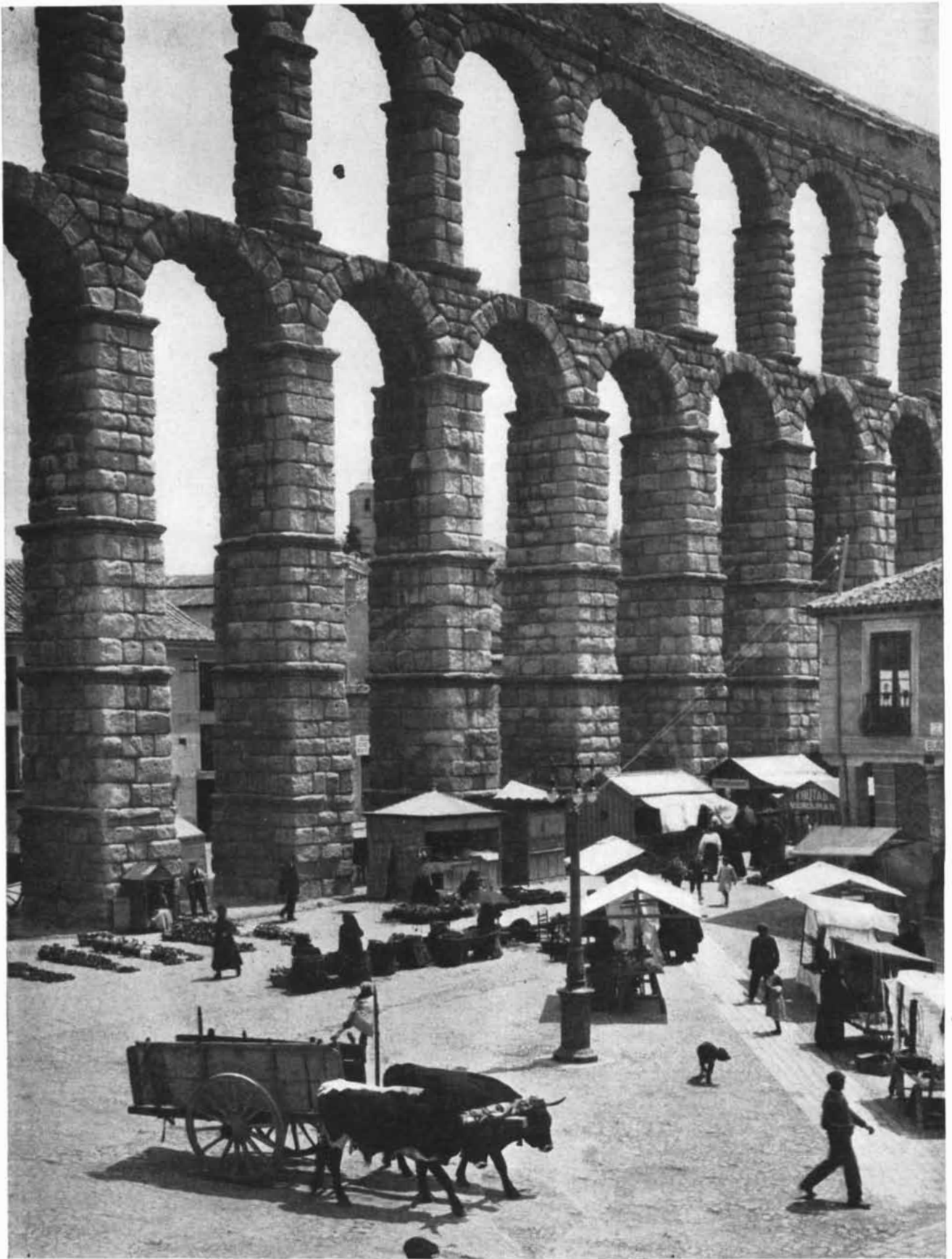
ROMAN AQUEDUCT in the Spanish town of Segovia was built during the reign of Augustus (27 B.C. to A.D. 14). Made of granite
