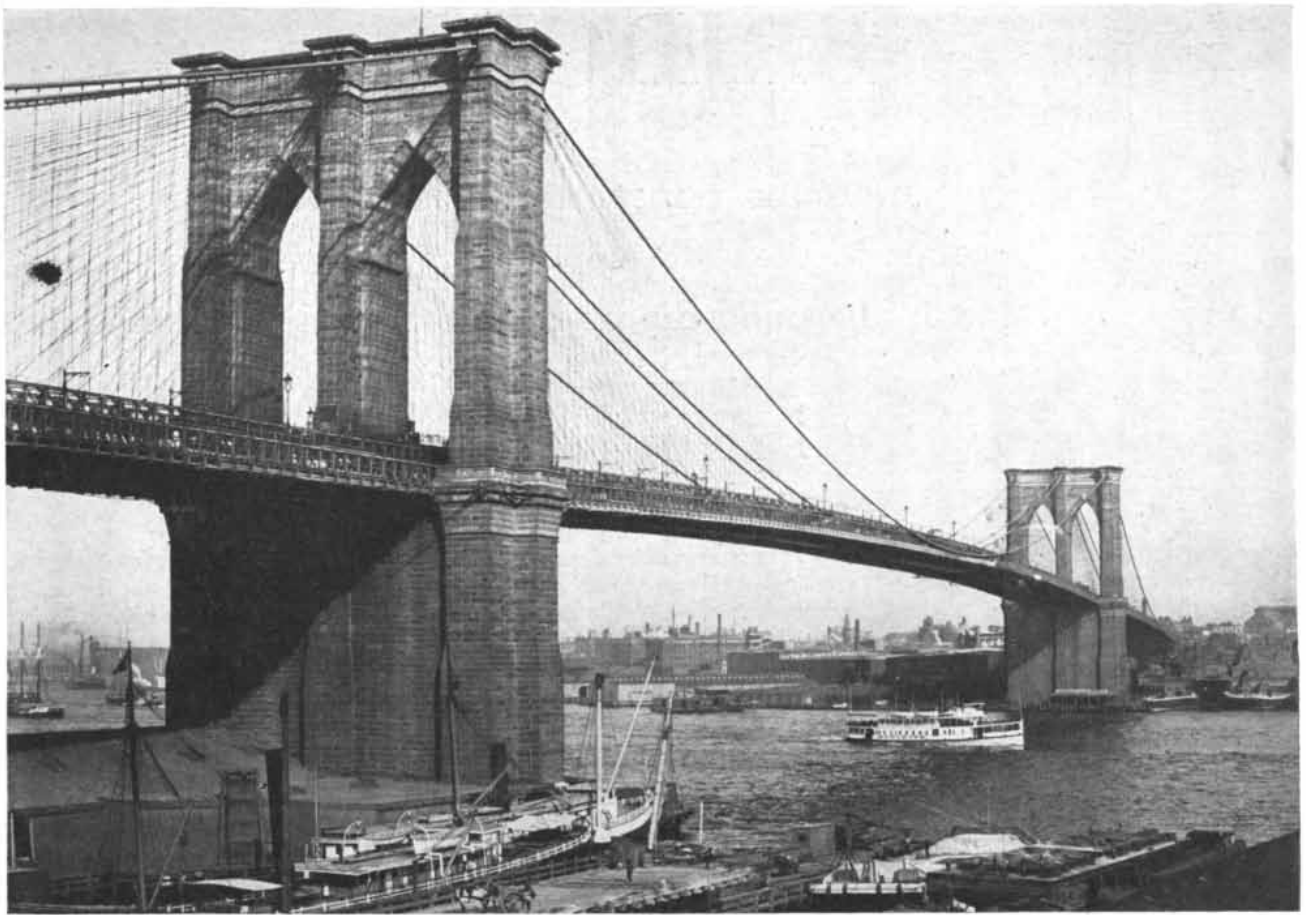
BROOKLYN BRIDGE was the first suspension bridge in which steel wire was used for the cables and steel members for the suspended structure. Its main span is 1,595 feet long. It was opened in 1883 and remained the longest bridge in the world for 20 years.
