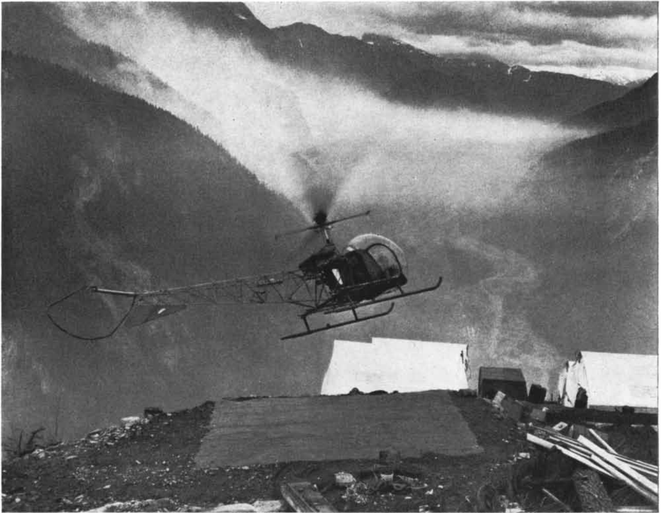
BELL 47D HELICOPTER takes off from a mountain camp of the $500-million hydroelectric power project of the Aluminum Com-
