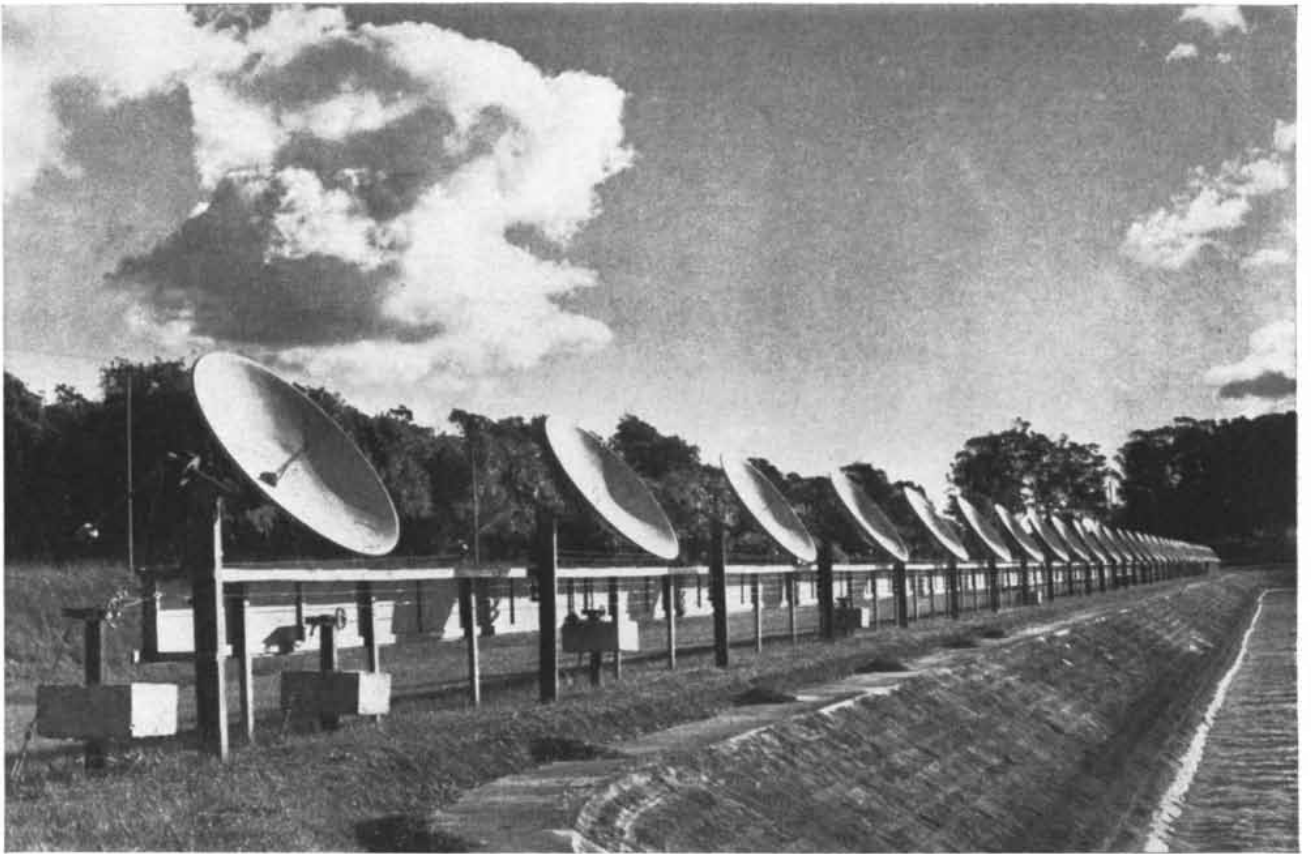
Radio interferometer at Sydney, Australia, has a 700-foot array of 32 parabolic reflectors.
