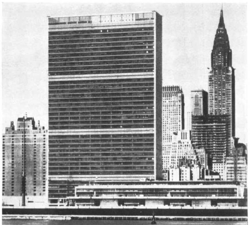
UNITED NATIONS SECRETARIAT building dominates Manhattan's eastern shoreline. Its glass walls are double-paned to provide insulation and are tinted green to reduce glare.
