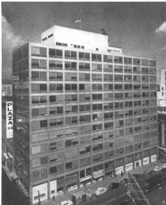
EQUITABLE LOAN BUILDING , built in 1948 in Portland, Ore., was the first skyscraper to incorporate a non-masonry curtain wall.
