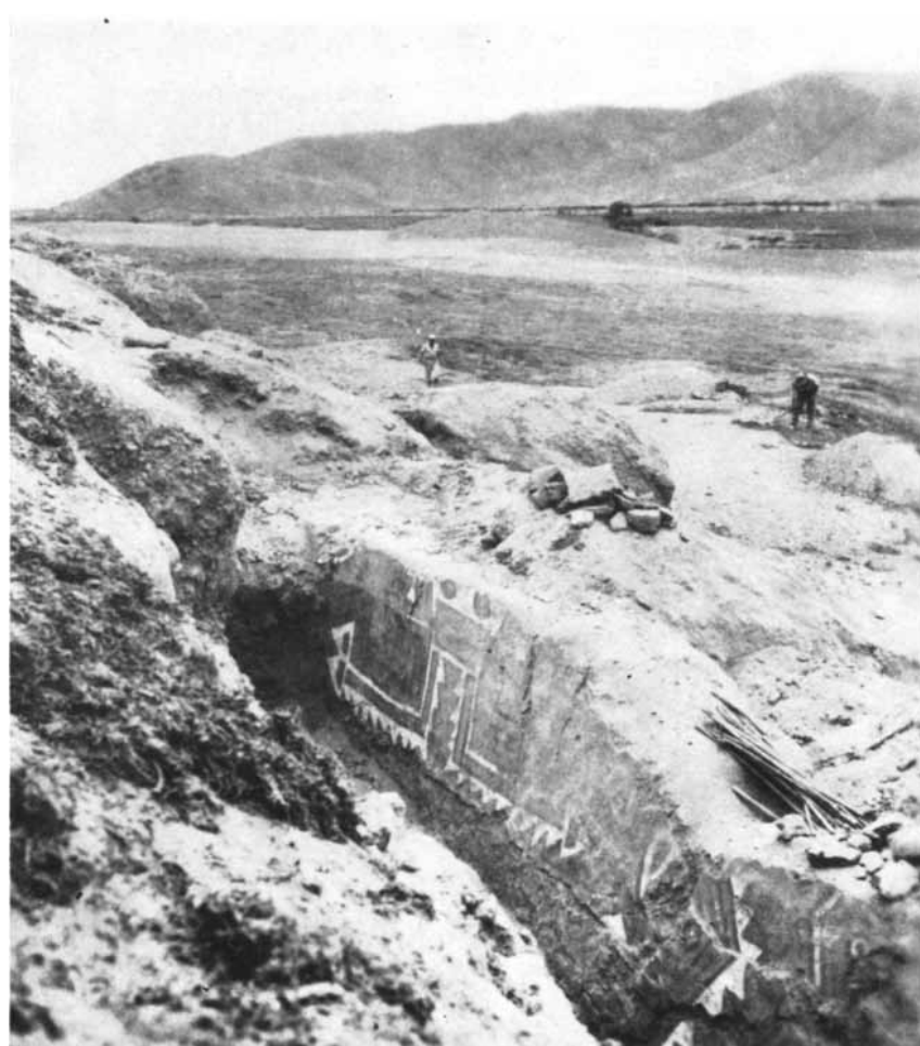
WALL PAINTINGS of the Cerro Culebra temple may be seen on the side of the trench in the foreground. The canes and adobe fragments at the right are remnants of the roof.
