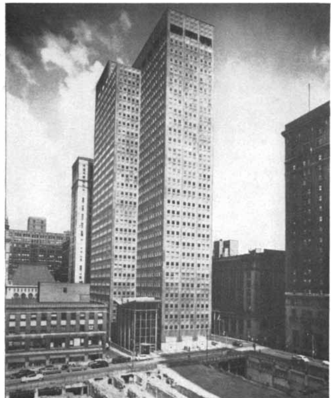
ALCOA BUILDING in Pittsburgh illustrates the present tendency away from all-glass walls in favor of prefabricated metal sections.
