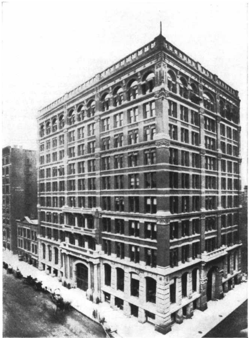
HOME INSURANCE BUILDING, built in Chicago in 1883, was the first skyscraper which had a separate steel skeleton and a curtain wall. It was designed by W. L. B. Jenney.
