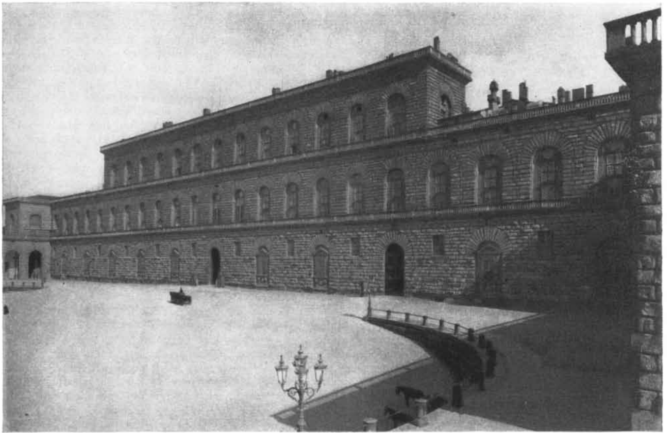
PITTI PALACE in Florence is a classic example of load-bearing wall architecture. Its walls are six feet, six inches thick. This
