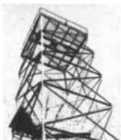
This 75 foot winch test tower is capable of simulating flight conditions and loads up to 30,000 lbs.
