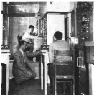
Inside this mobile ground station, test flights of the Avro Canada CF-100, RCAF all-weather interceptor for continental defense, are "seen" and "heard" with magnetic tape recorders.
