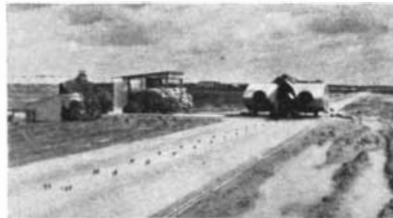
This jet-propelled test car was designed by AAE for the development of arresting gear and barriers.
