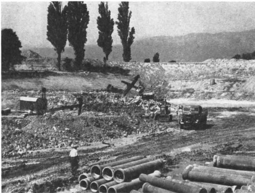
SITE OF CERN, the European center for nuclear research, was visited by many delegates interested in the international project. The excavation is for the magnets of the 600-million-electron-volt synchrocyclotron, which are scheduled to be erected at Geneva this month.
