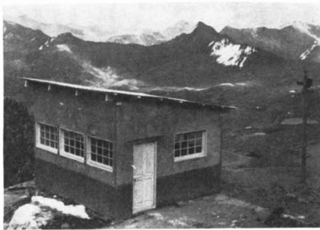
SAN NICOLAS STATION of the Institute is a small building for occasional studies of miners who work nearby at 16,500 feet.
