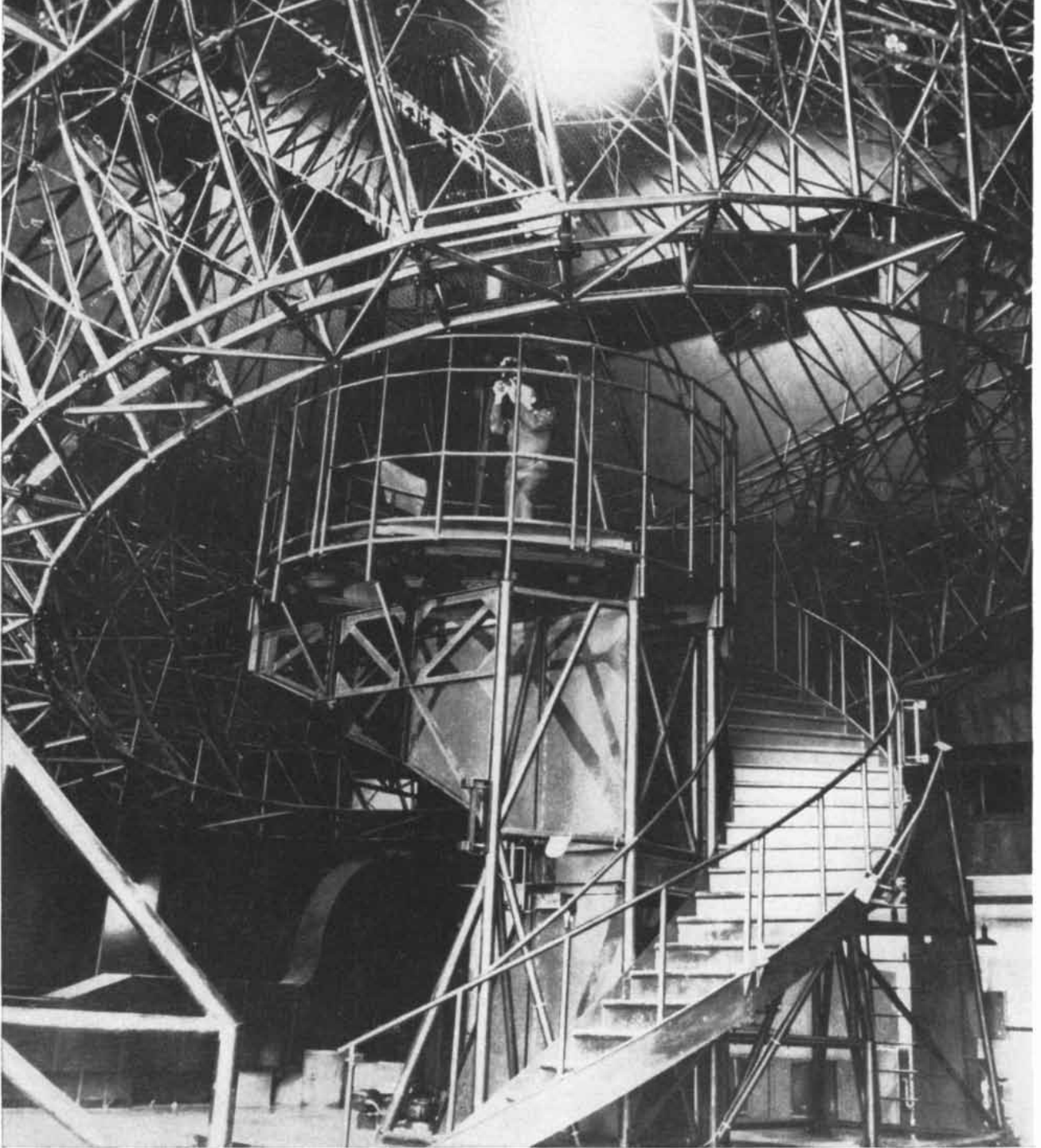
CELESTIAL NAVIGATION —Link Aviation's high-speed, high altitude celestial navigation trainer; only such trainer capable of simulating trans-Polar flight. Trains navigators in techniques of guiding planes by the stars.
