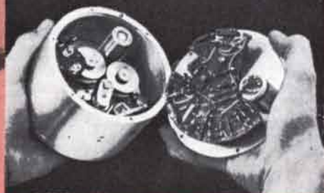
GLENNITE MODEL KAT-1 SELF-RECORDING ACCELEROMETER
