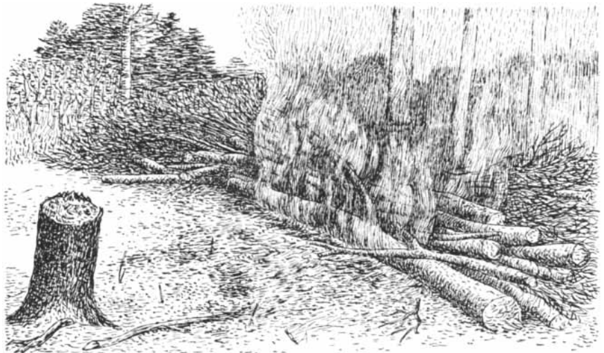
TREES WERE BURNED by covering them with brushwood and igniting a 30-foot strip. When the strip was almost burned out, the larger logs were used to light the next one.
