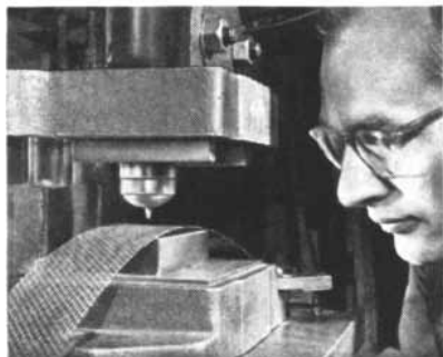
Forming and cutting the concave-convex spring from "BERYLCO" brand #25 wire cloth.
