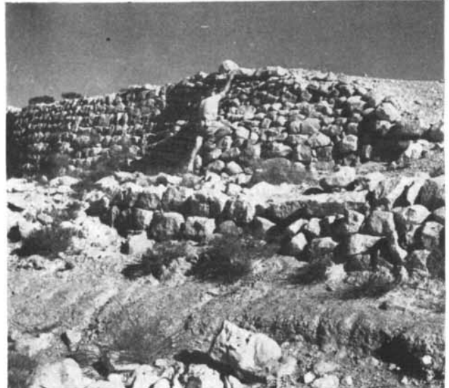
The bottom of the dam is built up in steps. The photograph at the right shows a relatively high wall which kept water in the wadi.
