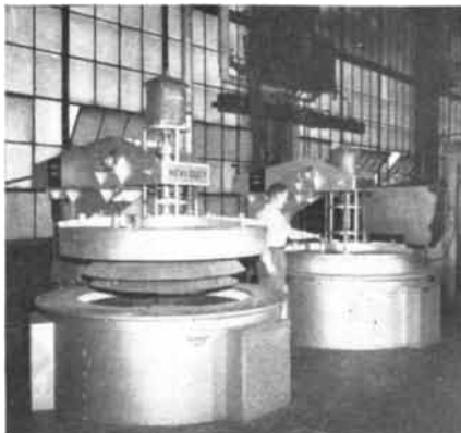
Part of the battery of electric heat-treating furnaces at CPT. Pieces up to 13 feet long can be handled in these furnaces and quench tanks.
