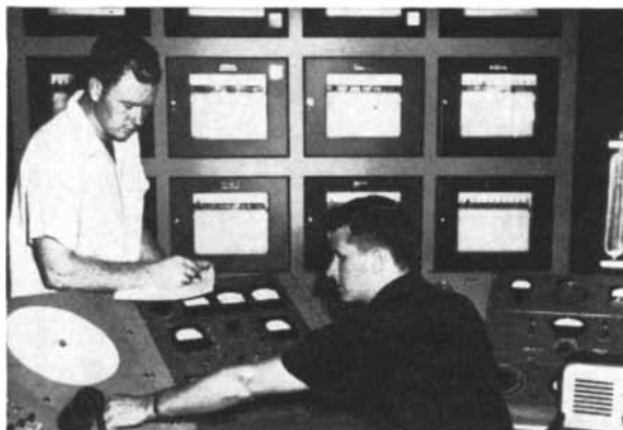
Honeywell control instrumentation for the first privately owned reactor, at North Carolina State College.
