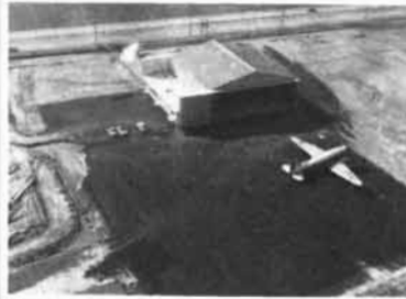
Initial unit of flight test facility
