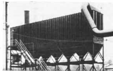
Fabric in Dracco Multi-Bag Filter cleans air at Jones & Laughlin Plant
