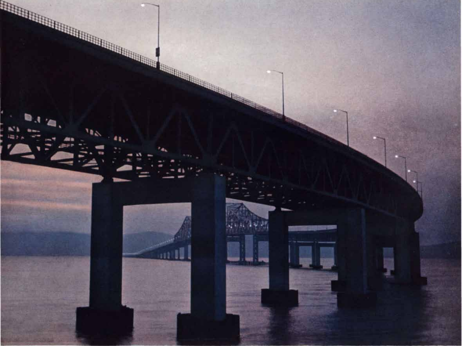
The New York State Thruway curves gracefully across the Hudson River just north of New York City on the new 16,000-foot Tappan Zee Bridge.
