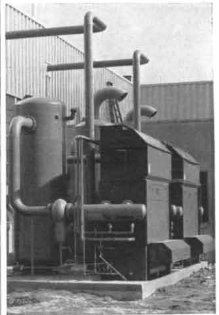
This Niagara Aero After Cooler also cools compressor jacket and intercooler water.
