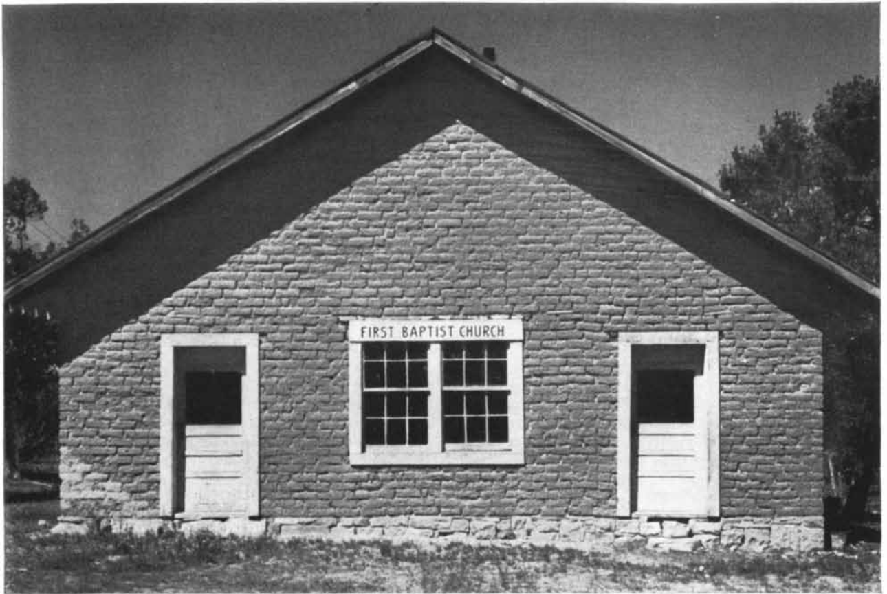
TEXAN HOMESTEADER CHURCH is one of 10 to which 250 homesteaders in the Gallup region belong, and is a cruder structure
