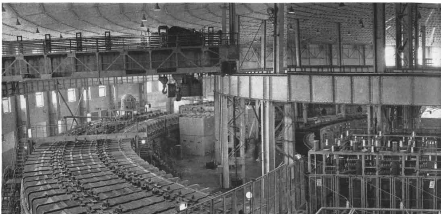
10-BEV PROTON SYNCHROTRON is nearing completion at the Central Institute of Nuclear Research at Bolshoya Volga near Mos-
