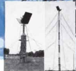
Transportable 800 lb. Magnesium antenna mast telescopes to 100 ft. Trained crew of 8 men can erect mast in less than an hour.
