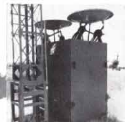
Microwave System capabilities include the transmission of voice communications (up to 72 two-way channels), radar data and radar control functions.
