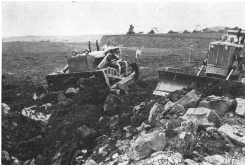
WORKED-OUT COAL MINE in Ohio is graded by bulldozers in first step toward reclamation of land. This strip mine was worked by power shovels. Grading will reduce erosion.
