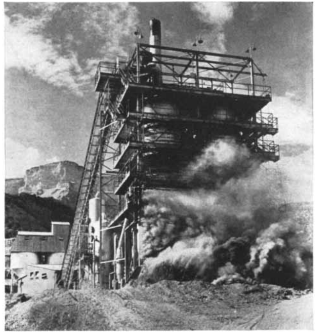
OIL-SHALE ASH , making a dust cloud at foot of the retorting plant, presents a major problem of disposal. Even rich oil shale, assaying at 30 gallons per ton, yields a ton of ash per barrel.
