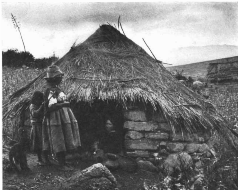
VICOS HOME has a circular wall and a conical thatched roof. Some two thirds of the Vicosinos live in such houses. The rest dwell in rectangular adobe structures with tile roofs.
