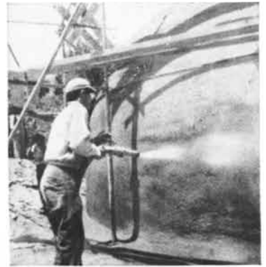
Final spraying of concrete on pneumatic form
