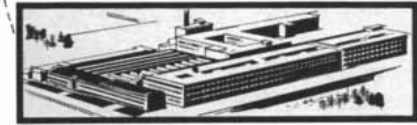
Buffalo Engineering Laboratory and manufacturing facilities for the Division occupy some 170,000 square feet of floor space in this industrial center. The Laboratory specializes in the development of advanced communications techniques and equipments.
