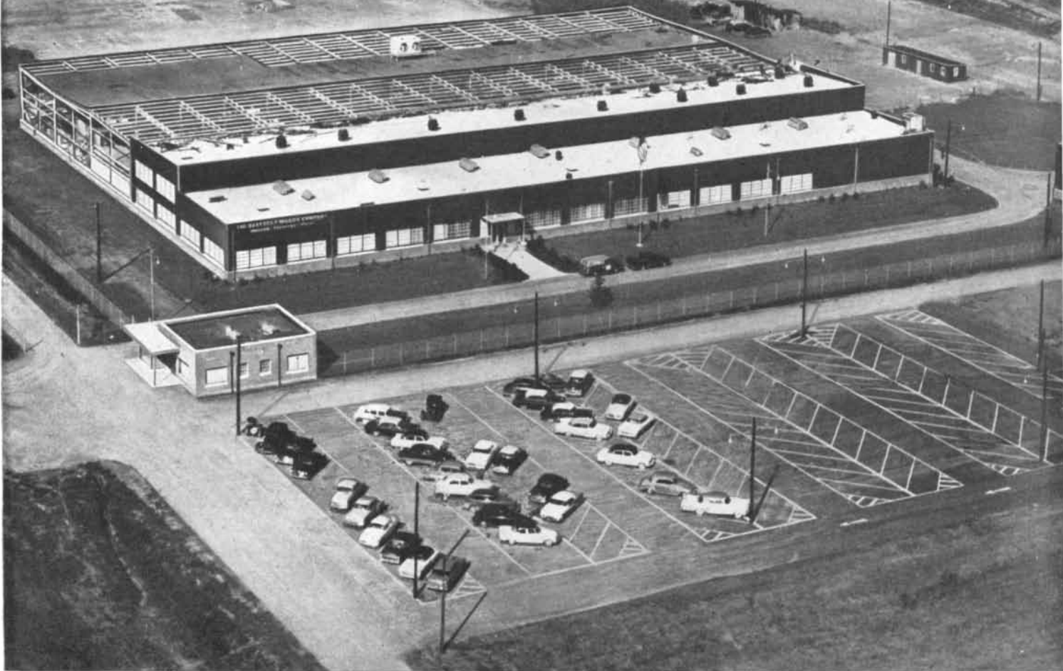
B&W Nuclear Facilities Plant in Lynchburg, Virginia, showing new expansion program under construction.
