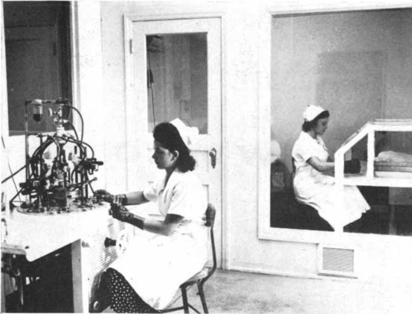
Ampoules are filled in DRY box at right and sealed in near room, held at 10% relative humidity by a Type CH Lectrodryer.
