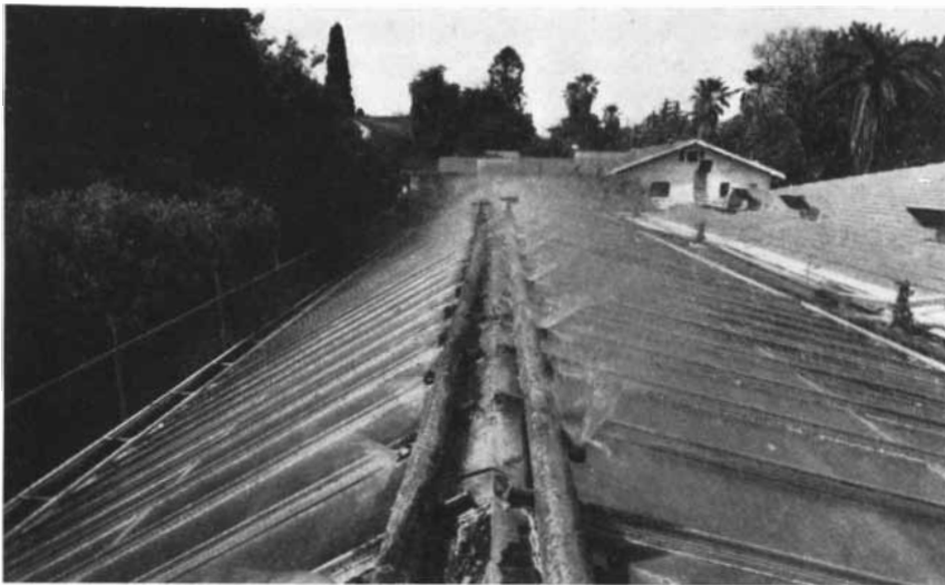
COOLING WATER is sprayed on the roof of a greenhouse in the laboratory. Most of the solar heat which accumulates in the greenhouses is removed by the rapid circulation of air.
