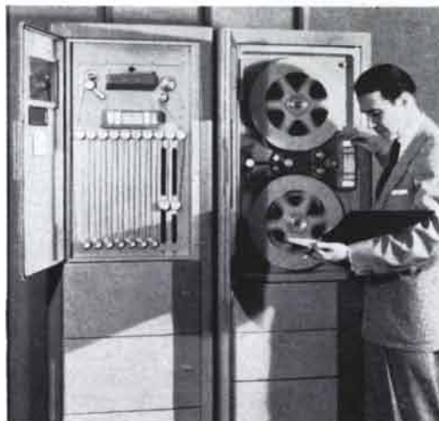
The new Ampex FL-100 Tape-Loop Recorder being used with an Ampex FR-100 Reel-to-Reel Recorder. Interchangeable plug-in units make the two compatible with any combination of track characteristics.
