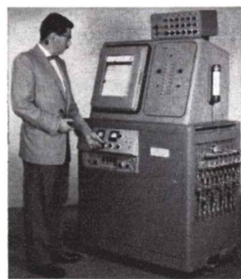
General Petroleum Corporation depends on a special Consolidated Mass Spectrometer to analyze combustion gases and control underground firing for oil recovery.
