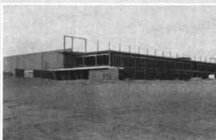
First unit of Denver manufacturing plant now nearing completion
