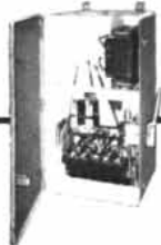
Bulletin 646 Manual Auto-transformer Starter.
