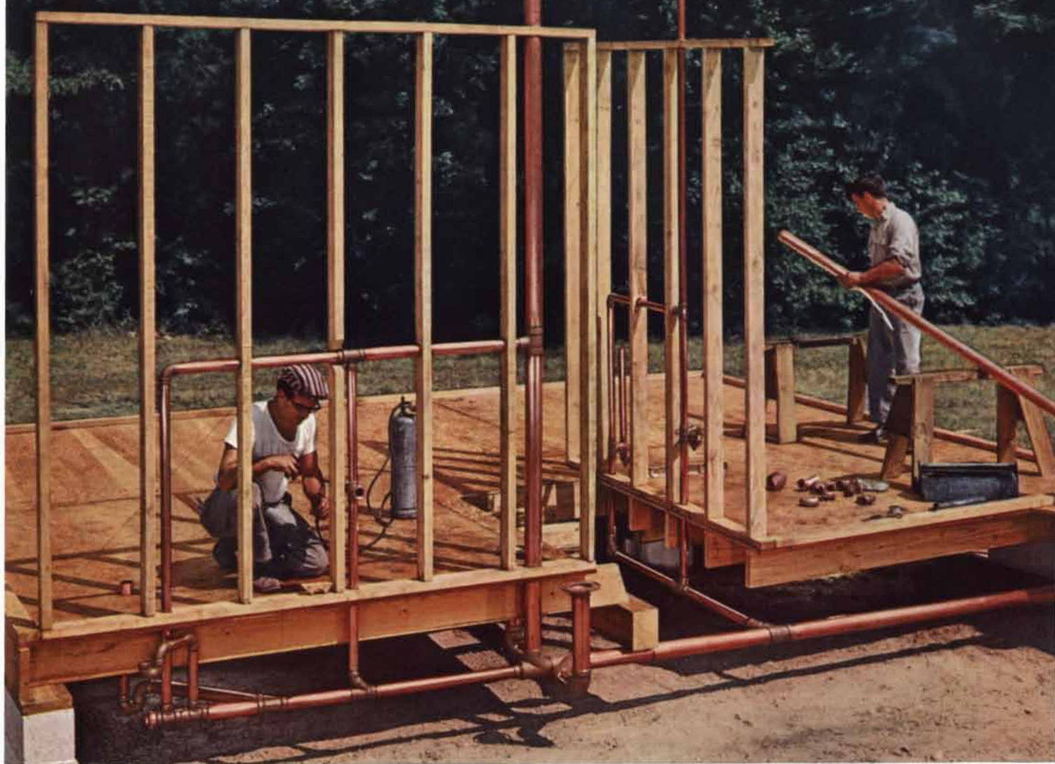
Model of a typical modern copper tube sanitary drainage system for a kitchen and two baths in a ranch-style home. Plumbing contractor (left) is shown making a solder connection, while his assistant (right) prepares to cut a 20-foot length of copper tube.
