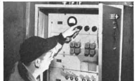
General Electric engineers, working closely with AL personnel, developed and installed the control systems which regulate the mill.
