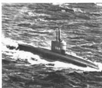
1957 Albacore, the sub that "flies" under water, has complete Sperry gyroscopic control system similar to an airplane's.
