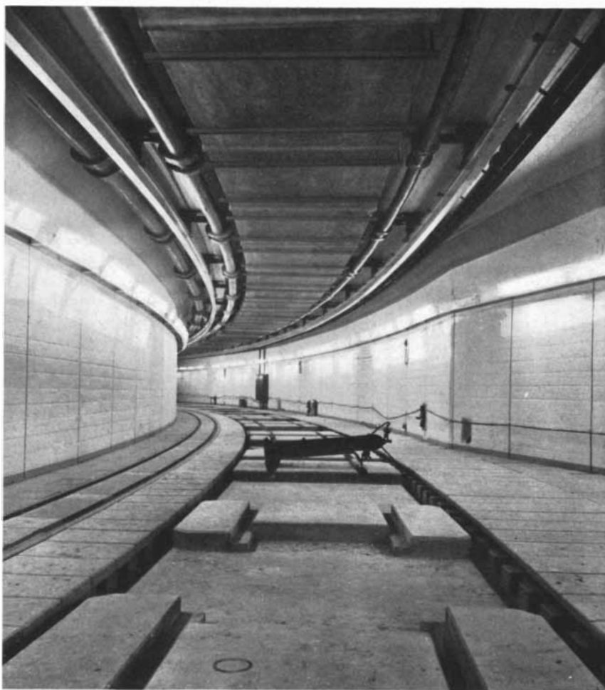
PROTON SYNCHROTRON IN GENEVA is designed to yield 25 bev. Shown here is a section of the interior of its ring building. This structure is approximately 660 feet in diameter.
