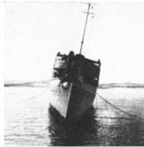
1913 First vessel automatically stabilized by Sperry gyroscopes was U.S. destroyer WORDEN.
