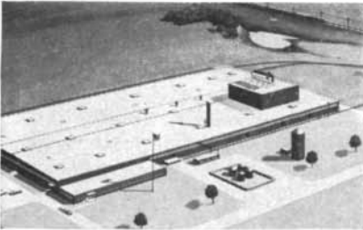
Wood Conversion (Weyerhaeuser Timber), Riverside, N. J.
