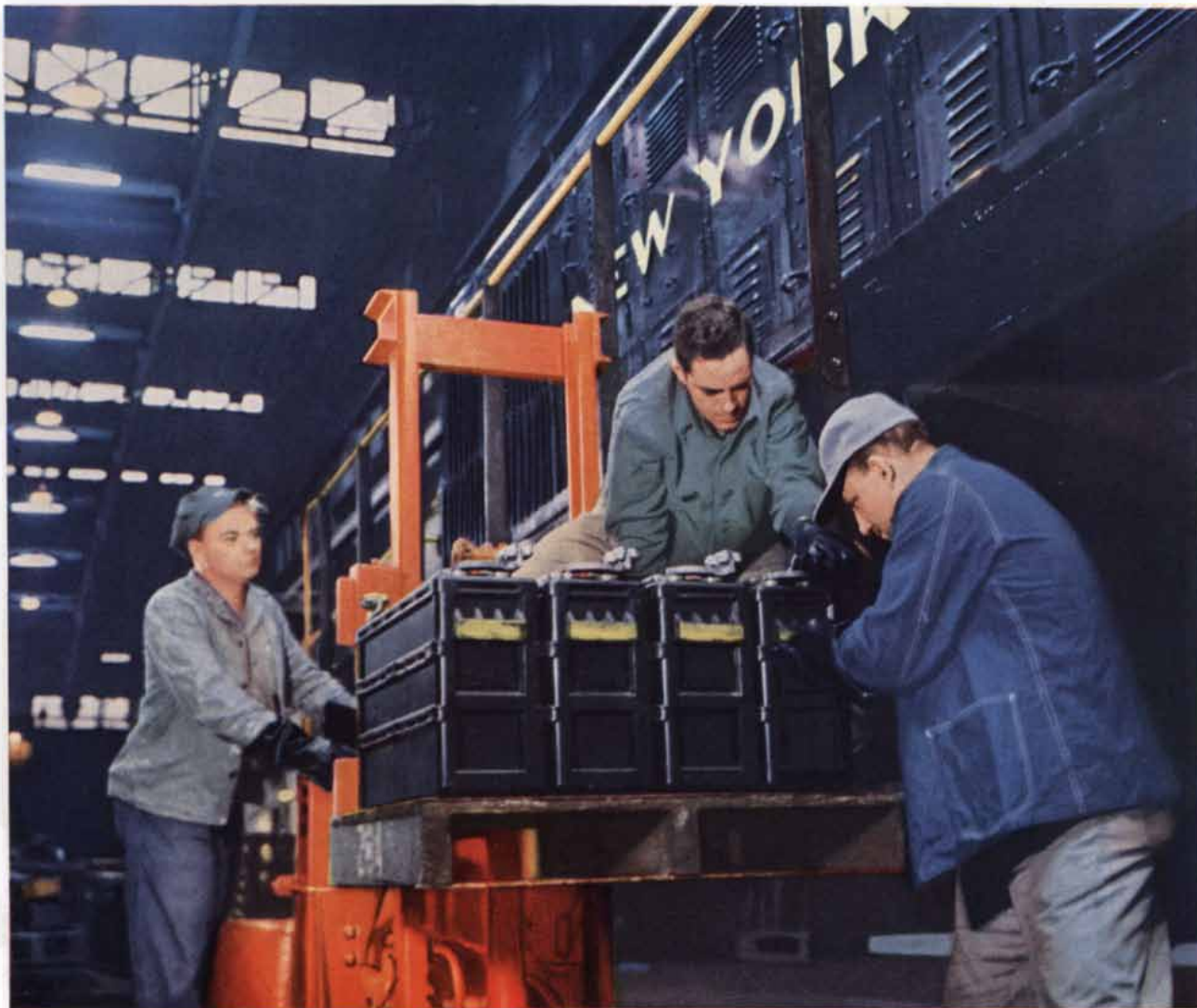
Photo courtesy Exide Industrial Division, Electric Storage Battery Co., Philadelphia, Pa.
