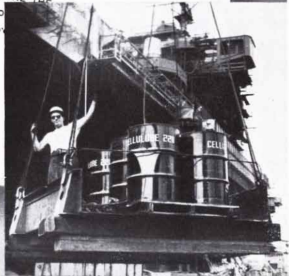
Fifty-five gallon drums of Cellulube 220 . . . part of a six-car trainload . . . being put aboard the new Independence. These hydraulic fluids will operate deck-edge elevators between hangar and flight decks.
