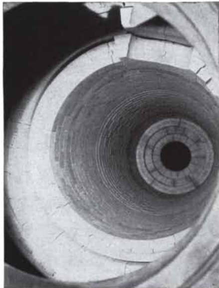
Newly Installed Pebble Heater at the Marquardt Aircraft Company of Van Nuys, California, designed to produce hot air for testing missile materials. Combustion Inlet shown above is lined with Norton Fused Stabilized Zirconia.
