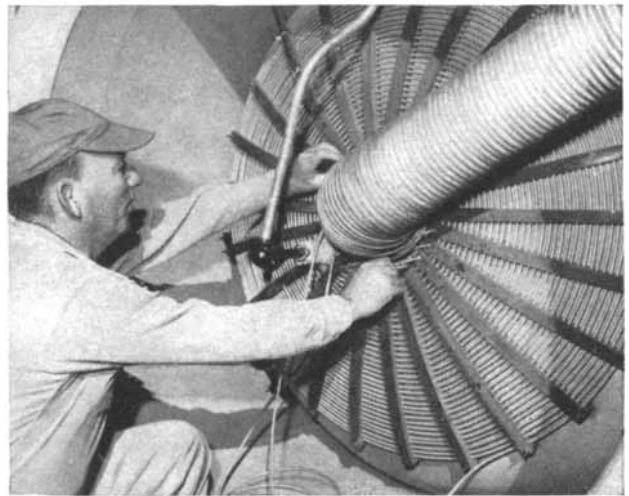
COPPER COILS being installed on the bottom of the main core vessel of the Organic Moderated Reactor Experiment.
