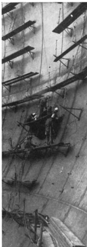
Interior of containment structure
