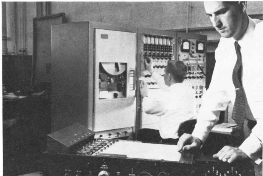
VIBRATION AND STRESS ANALYSIS data are obtained in hours instead of days with this special Westinghouse-developed Strain Gage Analyzer. From signals recorded on 14 channel magnetic tape, the analyzer plots multiple continuous curves visualizing vibration frequency and strain at varying engine speeds.
