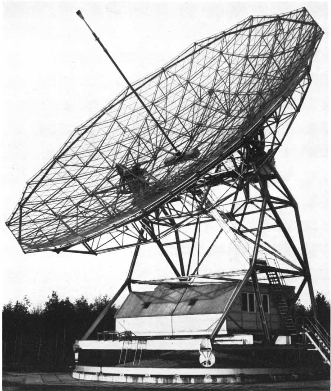
RADIO TELESCOPE that helped to determine the structure of our galaxy is located at Dwingeloo in the Netherlands. Its antenna and the first stages of its radio receiver are mounted atop the mast that juts from the face of the 82-foot reflector. The telescope framework
