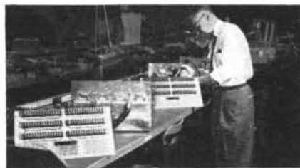
STANDARD MODULAR COMPONENTS are assembled on chassis mounted as individual drawers in relay racks. All drawers are connected by plugs for easy servicing.
