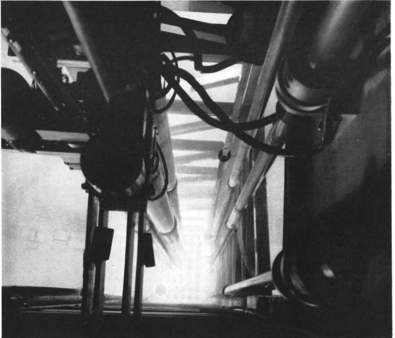
Curtiss-Wright Research Reactor Core—4 Megawatt
