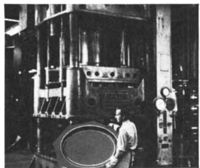
LARGE DRAW PRESS at Dow's fabrication plant forms magnesium sheet in one operation.
