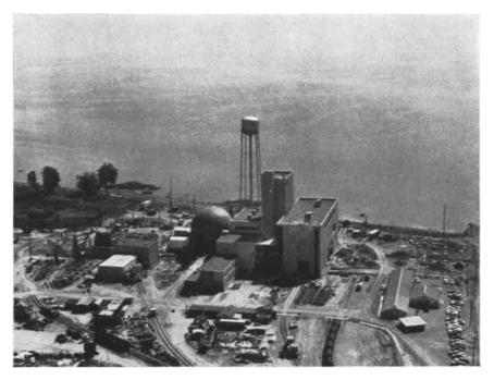
EXTERIOR VIEW shows the Fermi plant with Lake Michigan in the background. The steel dome that houses the reactor is 120 feet high and 72 feet in diameter. The adjoining buildings contain power-plant equipment such as heat exchangers and turbogenerators.
