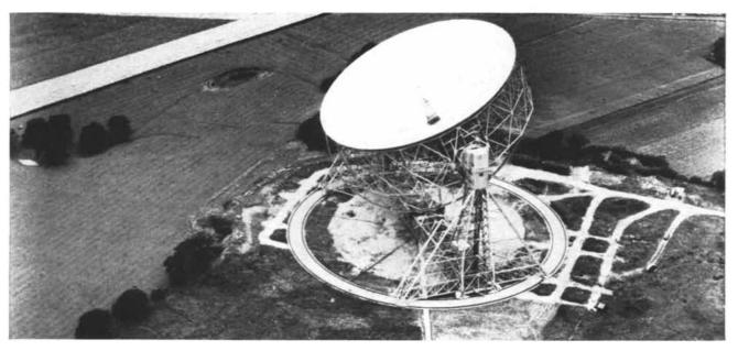
THE 250-FOOT TELESCOPE at Jodrell Bank in England is now the largest in the world. Its reflecting surface is steel sheets rather
