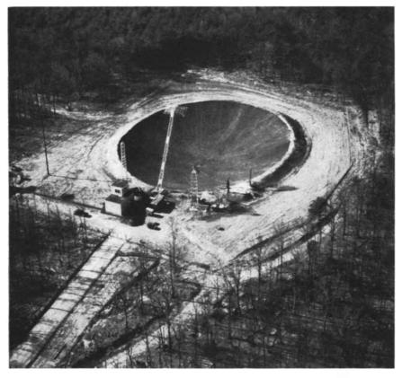
"HOLE-IN-THE-GROUND" ANTENNA devised by James H. Trexler bounces radar signals off moon. Paraboloid, 220 by 263 feet, is at Naval Research Laboratory station in Maryland. Large boom over surface moves to track the moon through restricted range.
