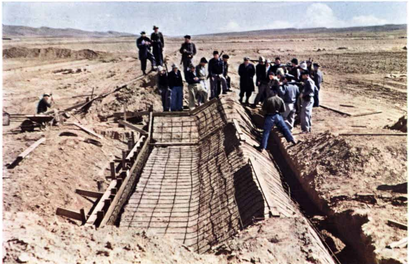
DESERT LAND in the Negev is made to support forage crops by diversion of flash-flood water, after methods employed by ancient Nabataeans. Water is trapped in basin fields, held long enough to
