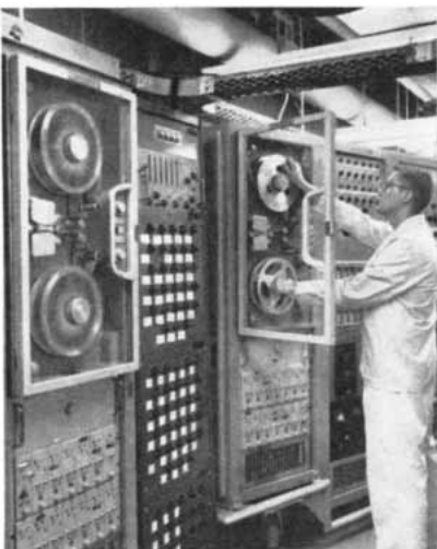
Test engineer removes fully-recorded reel of test data after switching all inputs to second transport without interrupting test.
