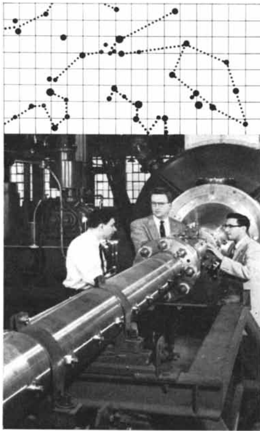
Six Inch Shock Tunnel and Large Air Arc Operated by MSVD's Space Sciences Laboratory
