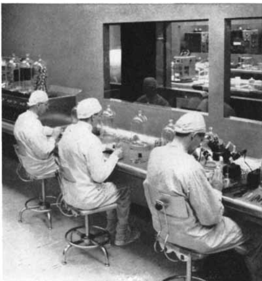
ENVIRONMENTAL CHECK FOR HUSTLER BOMB-NAVIGATION SYSTEM. The USAF's supersonic bomber must maintain global capability over a period of years. Here Sperry engineers put the control console of the B-58's rugged, highly accurate bomb-nav system through its paces.
