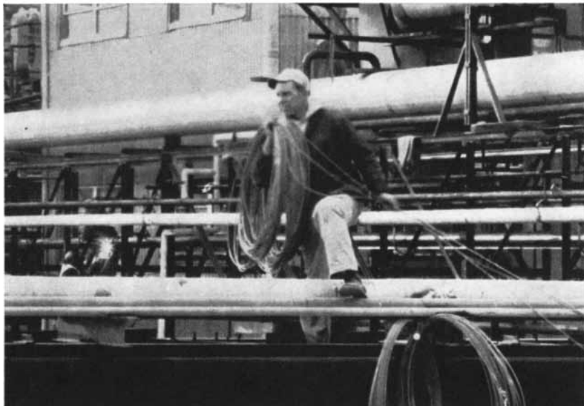
Installing PLASKON Nylon instrumentation tubing at Allied Chemical's Hopewell, Virginia plant. Note the 1000-foot, continuous, light-weight coils held by workman.
