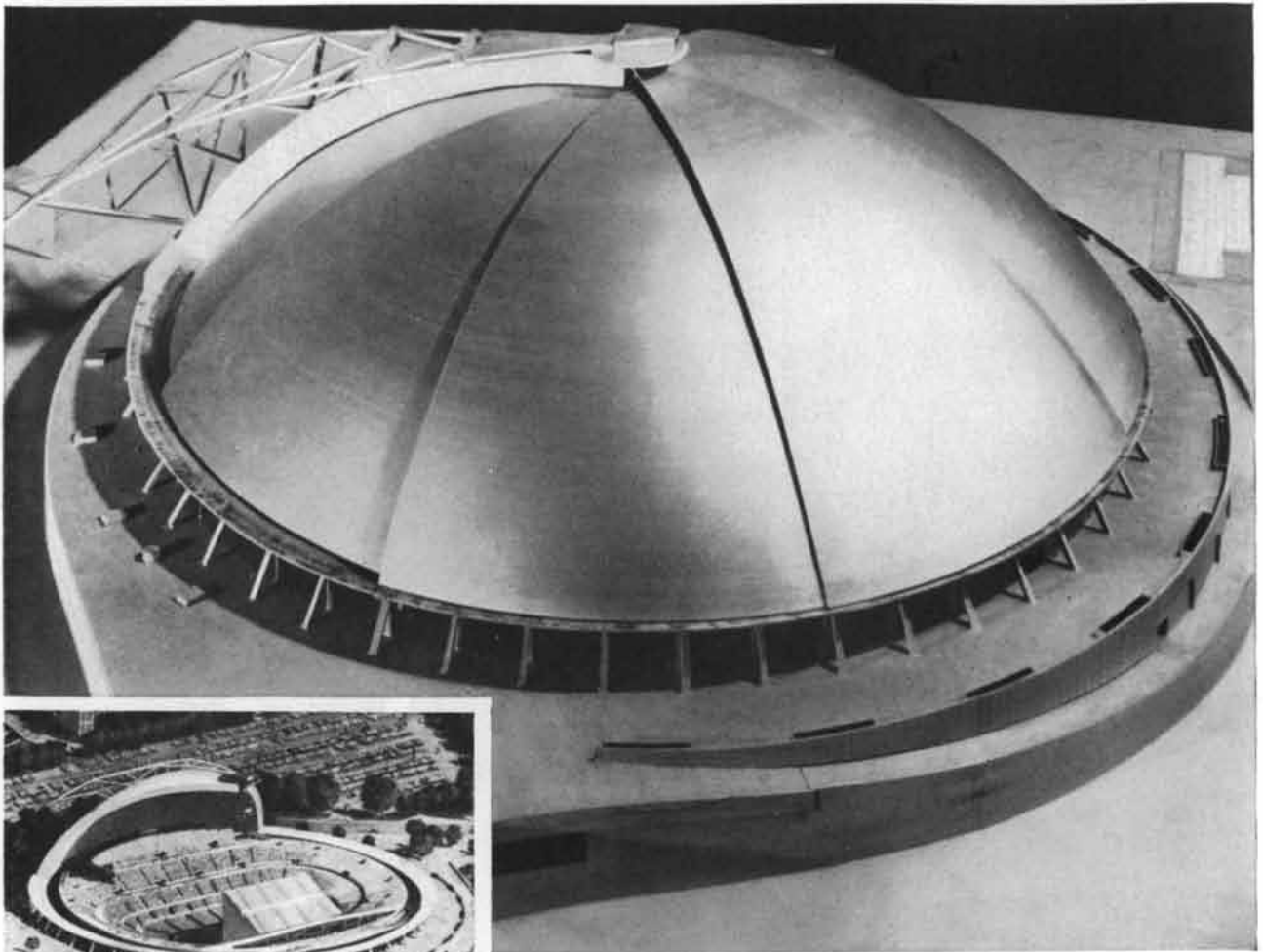
All-weather auditorium in Pittsburgh will be covered by a 415-foot diameter Nickel-containing stainless
