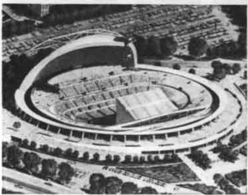
All-weather auditorium in Pittsburgh will be covered by a 415-foot diameter Nickel-containing stainless
