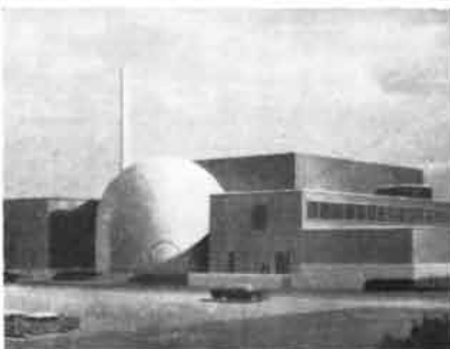
SOUTH DAKOTA: Architect's drawing of 66,000-kwe nuclear power plant with internal nuclear super-heat, now being designed for Northern States Power Company in cooperation with ten other midwest electric utilities.
