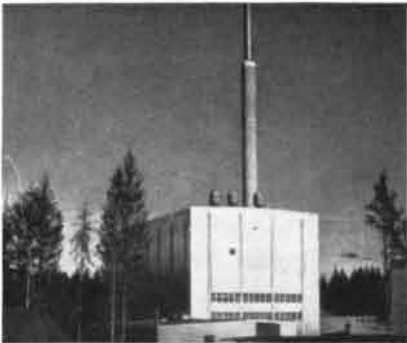
SWEDEN: New 30,000-kw research and materials-testing reactor for Atomic Energy Company of Stockholm.
