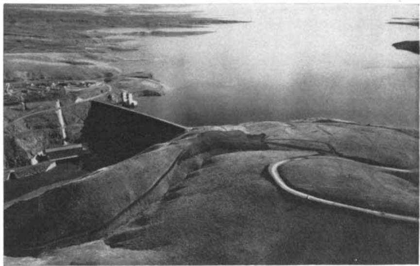
WATER FOR IRRIGATION, flood control and electric power is impounded behind Hirfanli Dam on Kizi Irmak river in Turkey. This 300-foot-high dam was completed in 1959.
