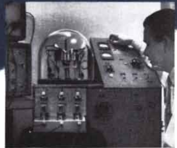
Bearingless support using electric fields
