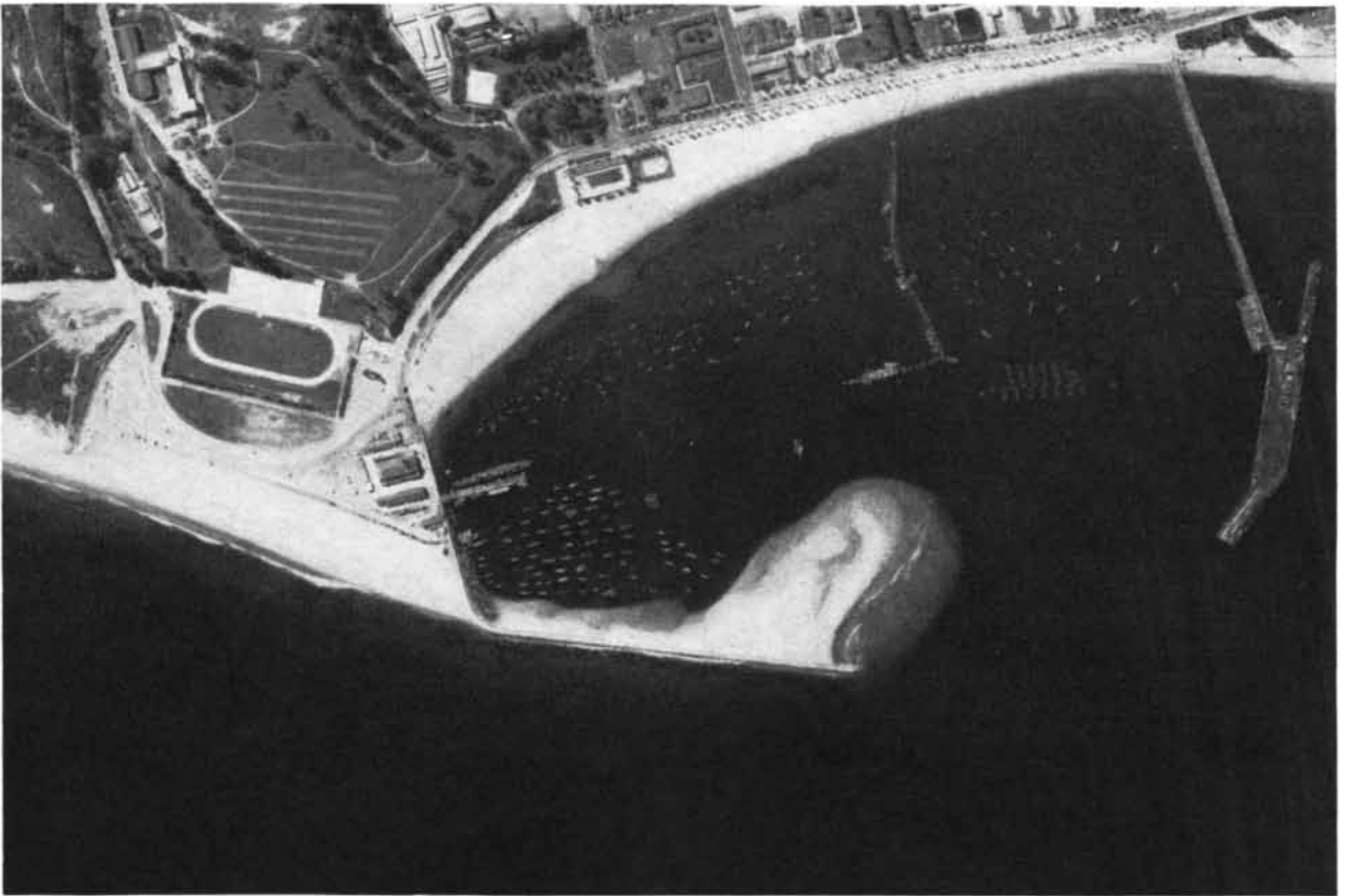
BREAKWATER AT SANTA BARBARA, CALIF., causes sand transported by a littoral current running from west to east ( i.e. , from left to right) to deposit in the sheltered water. A dredge in center of harbor moves sand beyond the large pier at right.
