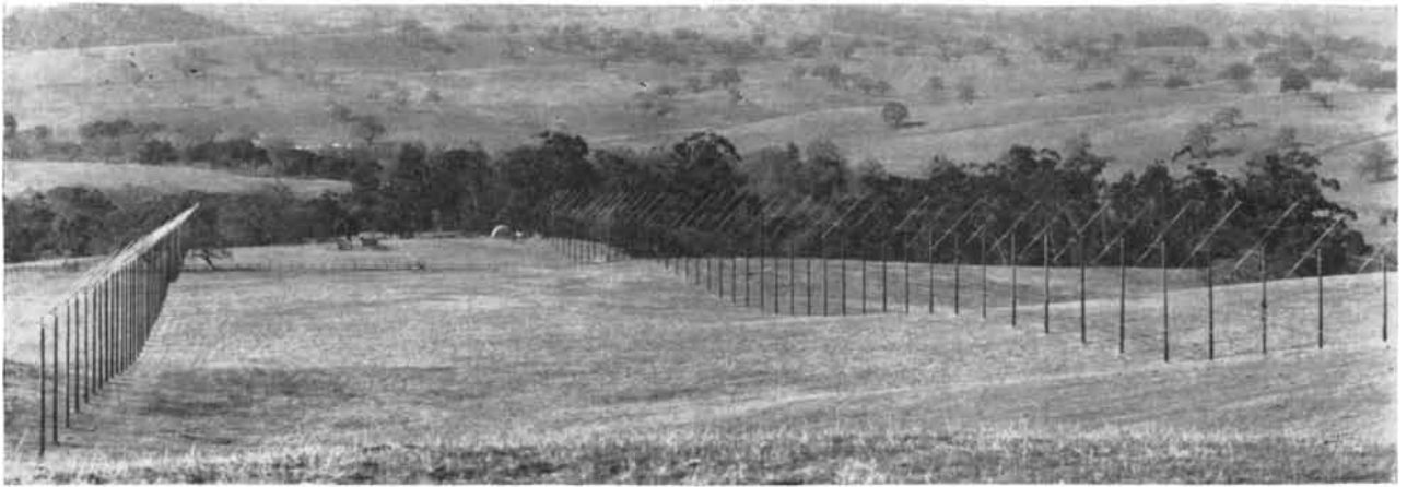
FIXED ANTENNA ARRAY at Stanford University is used to study meteors, the moon and the ionized gas between the earth and the moon. The array consists of wires and rods strung on poles in two 2,000-foot sections, and operates at a wavelength of 13 meters.
