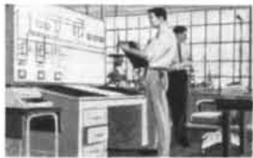
3. Instrumentation, control, and switching systems
