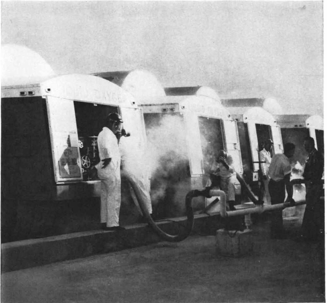
Pumping liquid oxygen for guided-missile fueling at Patrick A.F.B., Florida. Air Products, Inc., a pioneer in the production of LOX and other cryogenic materials, ships liquefied gases in these tank-
