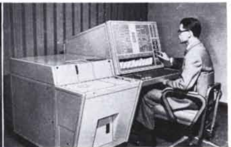
The Automatic Monitoring Console displays degradation and the location of degraded equipment.
