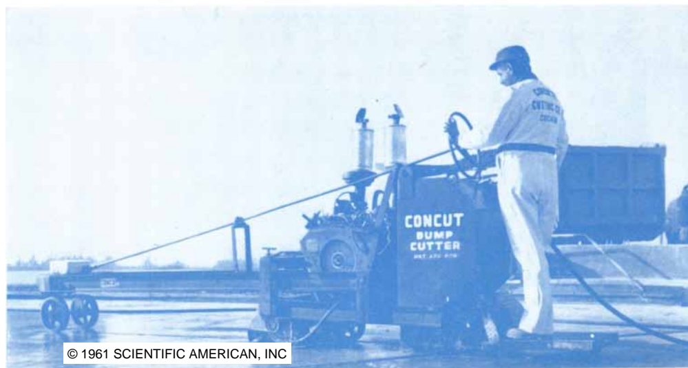
Diamonds remove bumps from concrete runways and highways
