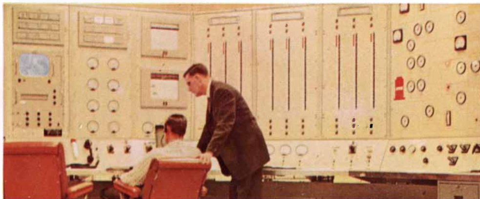
Master Control Room. This is focal point of the operating facility; providing remote indication of reactor performance and experimental conditions.
